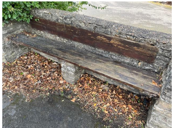
Wall of Queen's Head, King Edward Street
